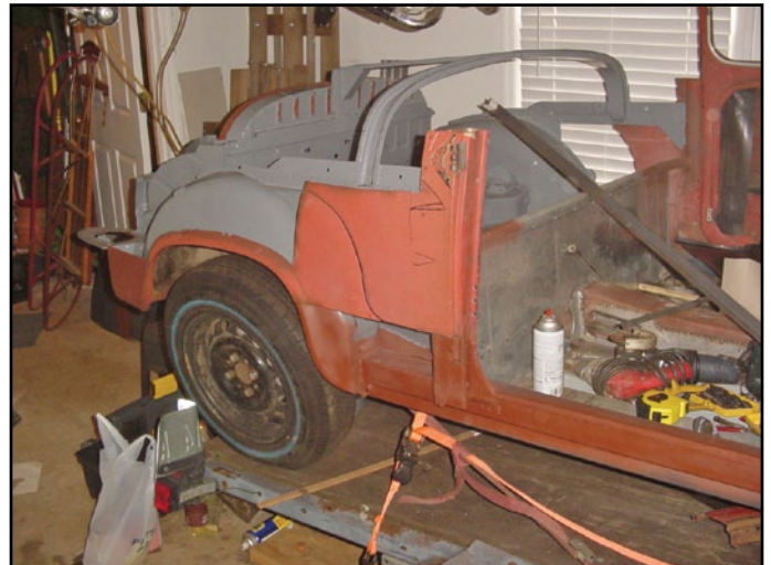
Prior to welding, body substructure is sandblasted, primed and painted.
